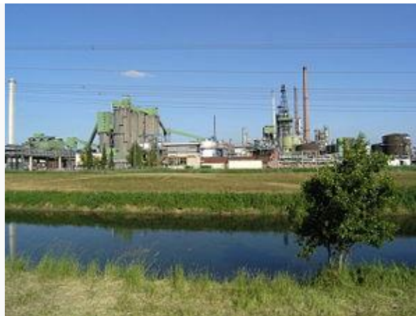
MiRO refinery at Karlsruhe
